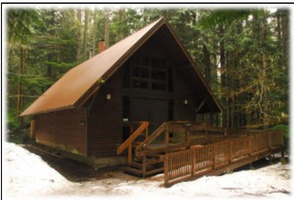
Slide Mountain Cabin - Ramp Access
