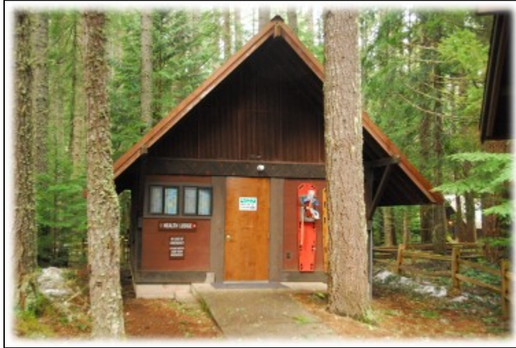
Women's Restroom/Health Lodge
